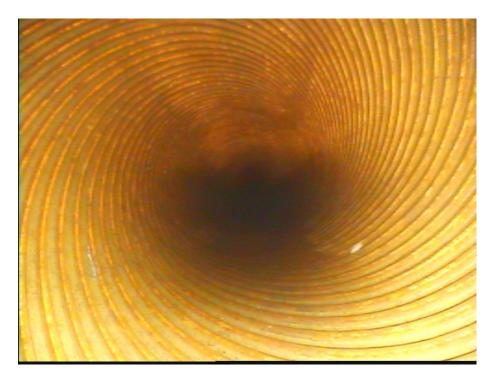
Boroscope Photos at Alfred Chiller #3 AFTER BallTech system installed
