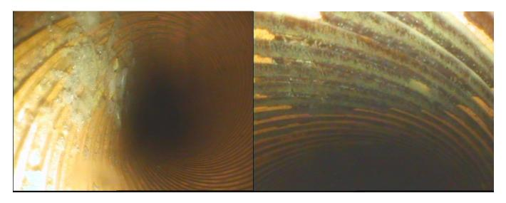
Boroscope Photos at Alfred Chiller #4 WITHOUT BallTech system installed
