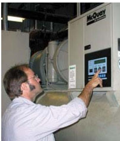
*Mark Hanson, service technician, finishes a maintenance job on a centrifugal chiller by verifying that actual conditions match performance specifications.*
